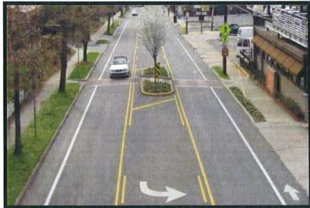
Figure 17. Median island providing pedestrian refuge on a three-lane section with center turn-lane. Source:
