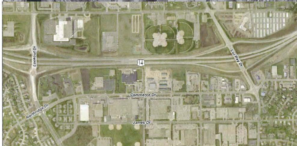
Figure 7. Commerce Drive Today – Realigned with Northridge Drive and almost fully developed carrying over 11,500 vehicles per day. Source: USGS, ESRI, Pictometry.
