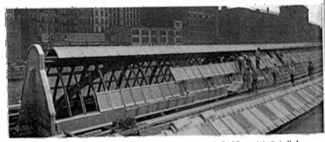
The Concrete Tile and Class Done Were Made to Fir Accurately to the Steel Frame of the Train Sheds.
