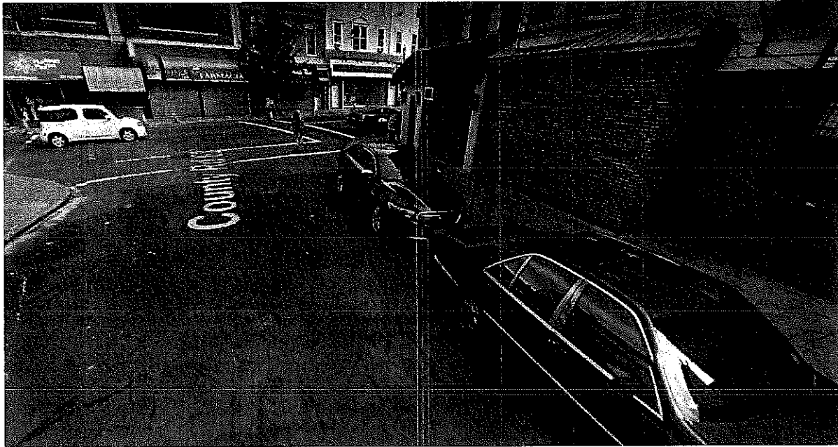
Figure 2. The intersection of Fairmount Avenue with Bergen Avenue has faded crosswalks, inadequate signage, and visibility issues that endanger pedestrian travel.
