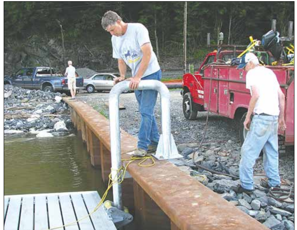
Matt Smith oversees the installation of the boat launch.
