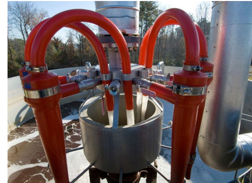
The addition of hydrocyclones for selective anammox bacteria retention (DEMON® process HRSD)
