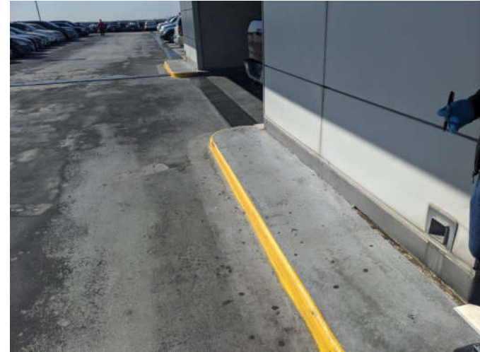
No. 2 View of yellow curb (Sample 2 Rooftop).
