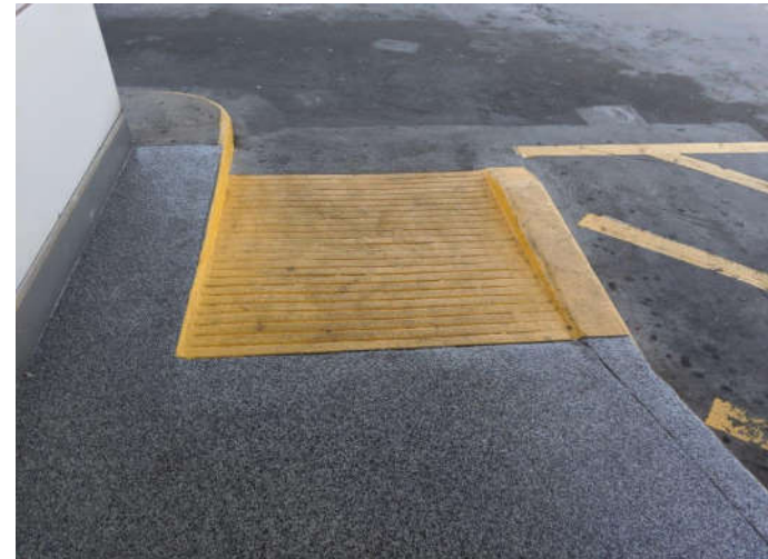
No. 4 View of yellow ramp (Sample 4 Rooftop).
