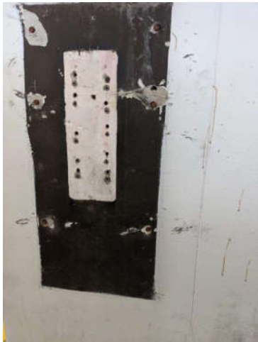
No. 25 View of the black wall paint (Sample 11 Level 3).
