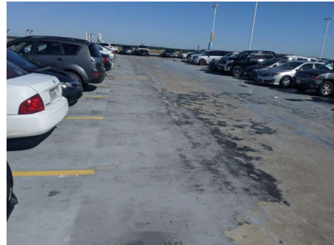
No. 14 View of gray floor paint (Sample 15 Rooftop).
