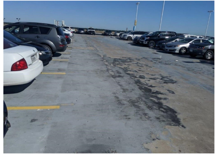
No. 2 View of roofing tar (Sample 2 Rooftop).
