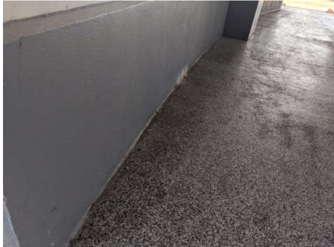
No. 13 View of gray wall paint (Sample 14 Rooftop).
