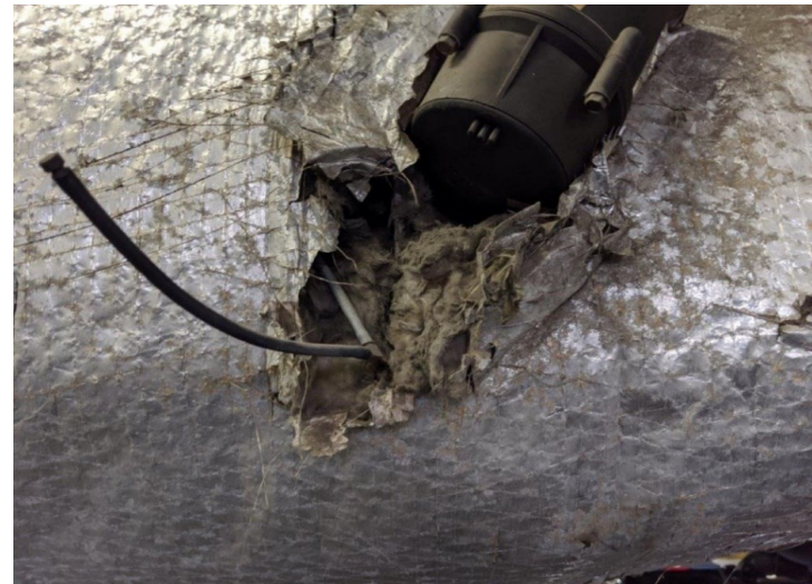
No. 8 View of exhaust insulation (Sample 4 Level 3).
