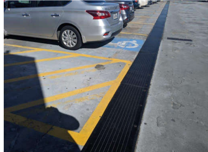
No. 6 View of yellow parking stripe paint (Sample 6 Rooftop).
