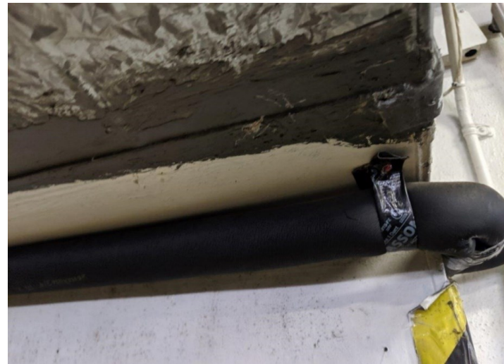
No. 6 View of air vent duct mastic (Sample 2 Level 3).
