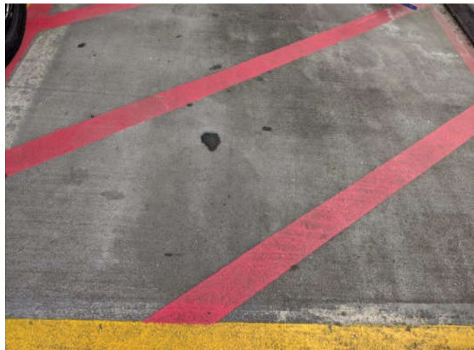
No. 29 View of red no parking zone paint (Sample 15 Level 3).
