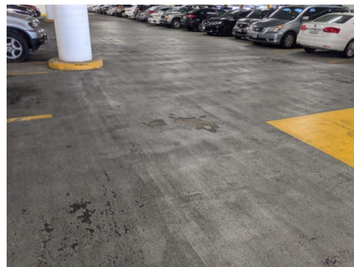
No. 24 View of the white column (Sample 10 Level 3).
