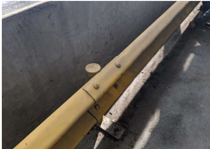
No. 17 View of yellow parking guard rail (Sample 3 Level 3).
