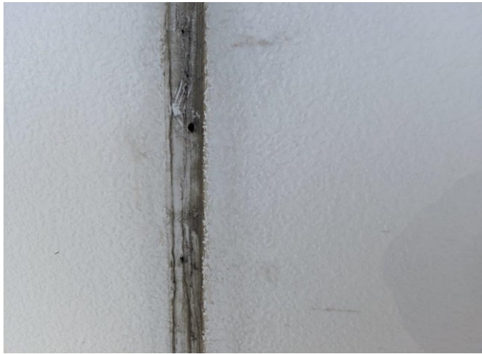
No. 1 View of building caulking (Sample 1 Rooftop).
