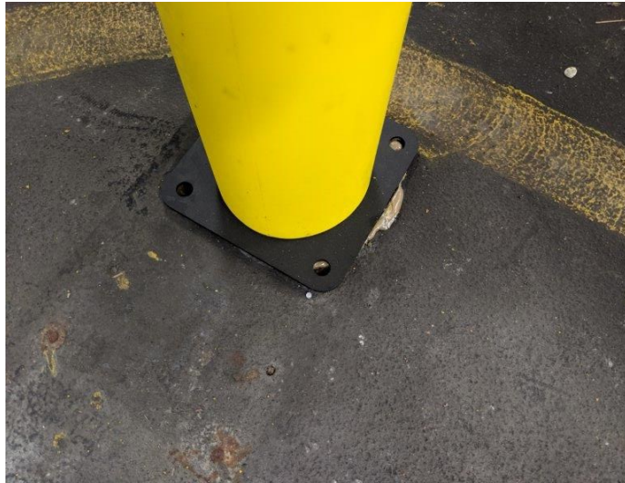
No. 9 View of handicap post base caulking (Sample 5 Level 3).
