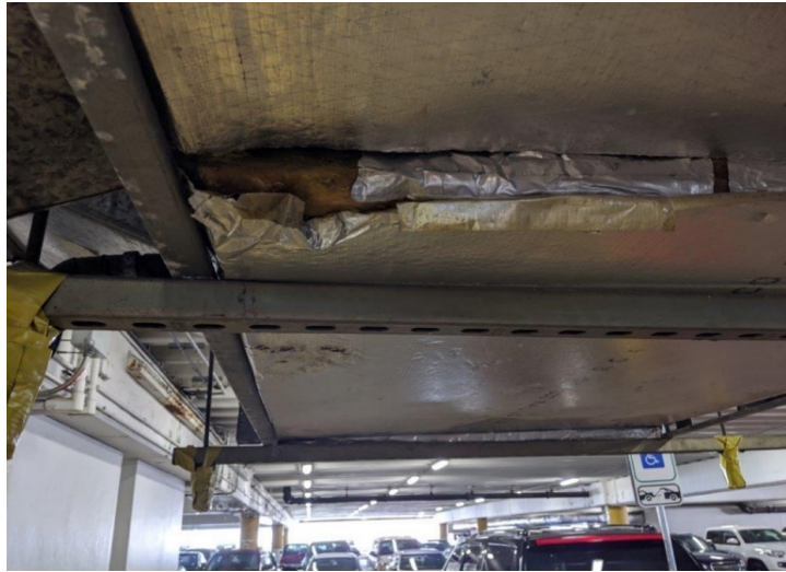
No. 5 View of air vent insulation (Sample 1 Level 3).
