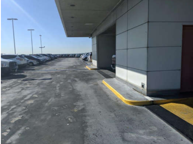
No. 1 View of the red door to far right (Sample 1 Rooftop).
