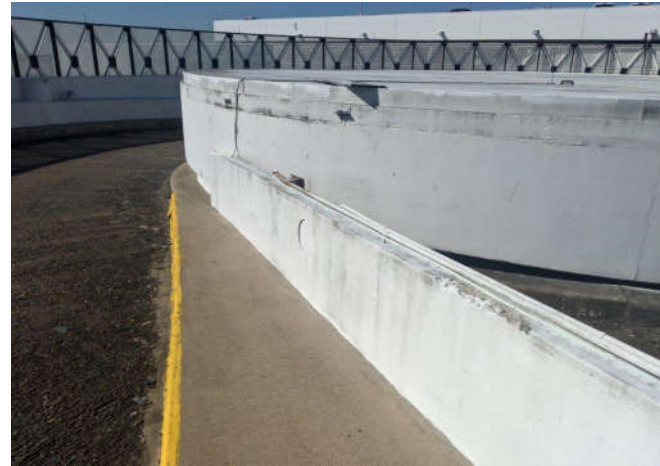
No. 10 View of white parking structure paint (Sample 10 Rooftop).
