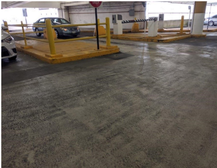
No. 7 View of flooring tar (Sample 3 Level 3).
