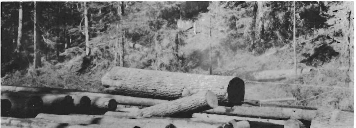
H. A. Peterson Large pine log being trailed in from the woods on the log chute at a landing on the Kalispell Creek Railroad. The wire rope (cable) attached to the tractor pulling the log is visible at the right, summer 1929.
