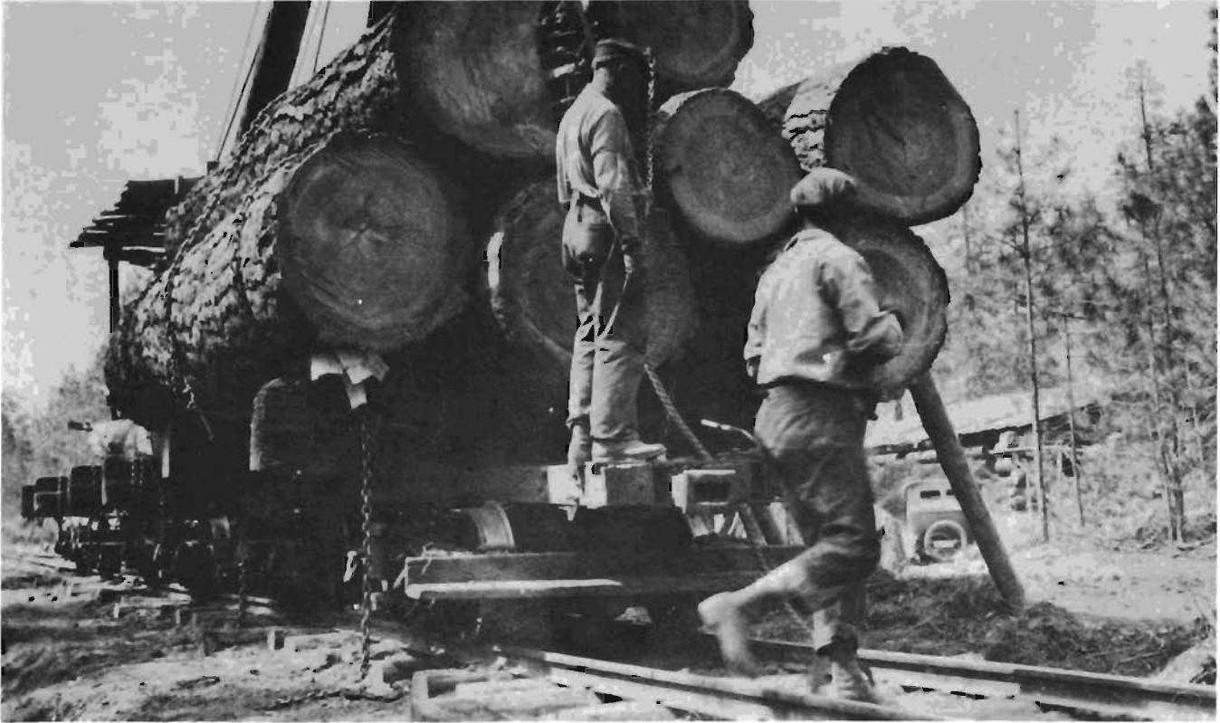
Two bunk log car being loaded by "home built" slideback log loader along Omak Creek during the fall of 1924. Loader rested on a rough skidder type sled built out of logs.
