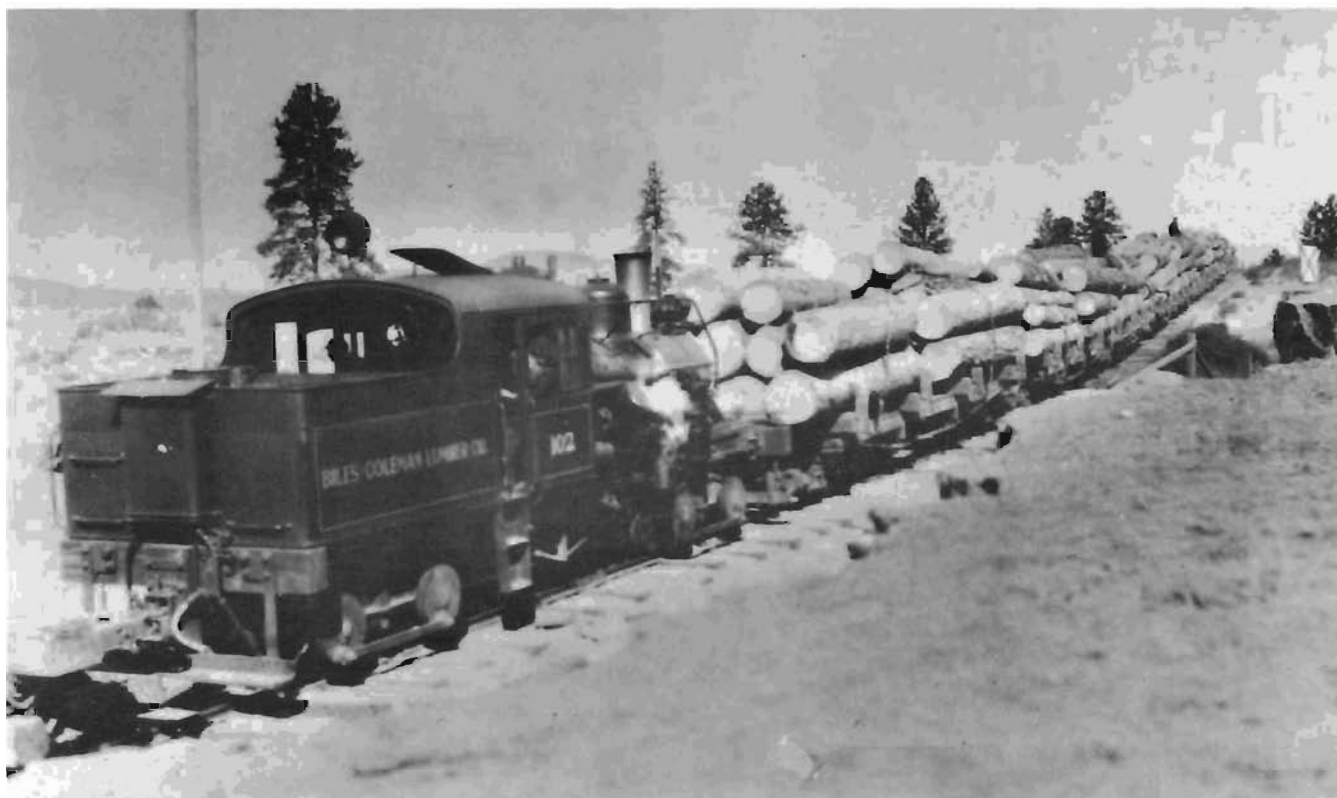
Biles-Coleman Lumber Company No. 102 and a loaded train of eight log cars drift down the 3.6% grade just to the East of St. Mary's Mission on the final leg of its trip to the mill, 1926.
