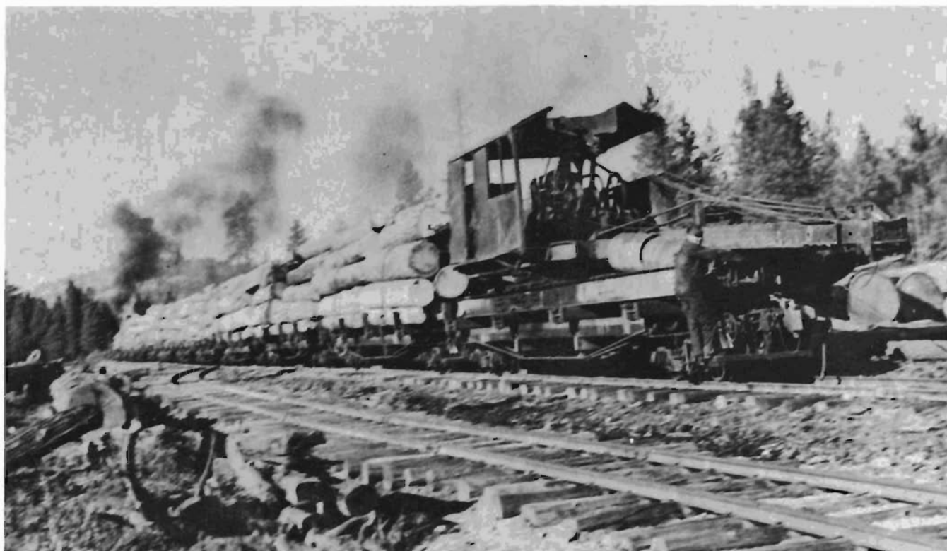
U. S. Indian Service Photo from J. E. Lewis Collection Loaded log train trailing a car carrying the loader with its boom lowered to allow movement over the main line leaves log loading landing No. 1.
