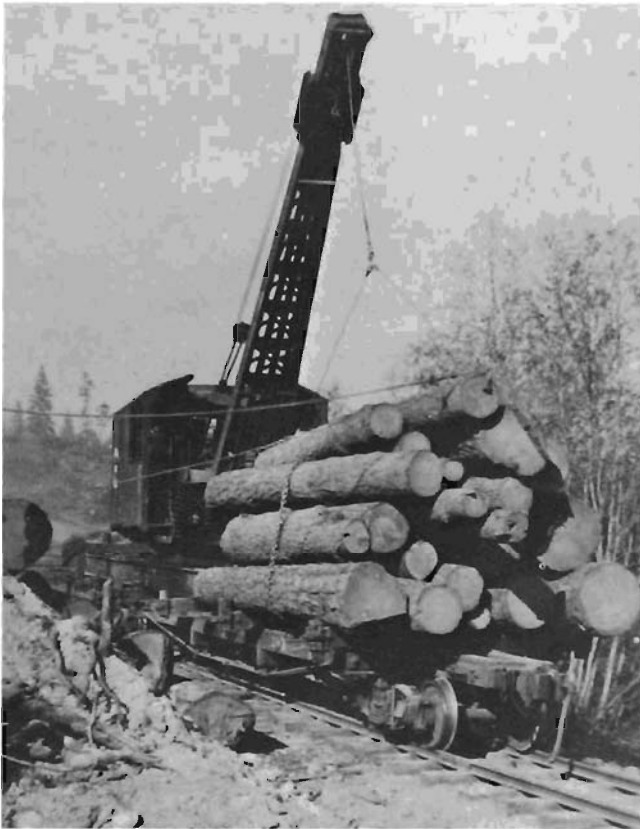
E. R. Aston Log car No. 101 being loaded with logs by the A. H. & D. log loader on the "A" line during 1927 after the original link and pin couplers had been replaced by automatic couplers.
