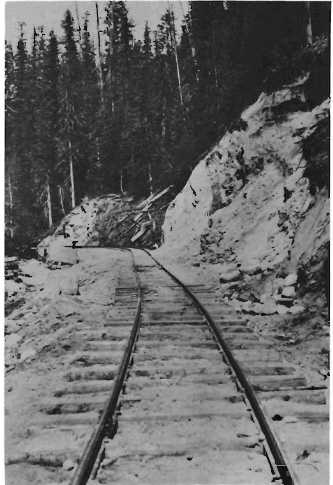
H. A. Peterson New narrow gauge track just built in a rock cut on the Diamond Match Co. narrow gauge railroad, spring 1930.
