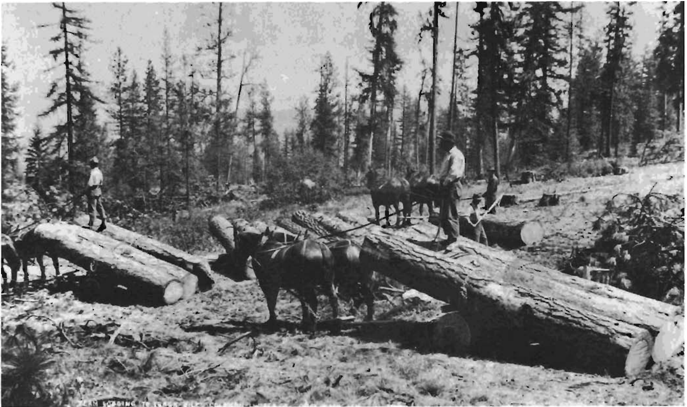
Ladd Photo from E. Aston Horse drawn dollies used to skid logs from the stump to rollways along the Biles-Coleman narrow gauge, "A" line, 1927.
