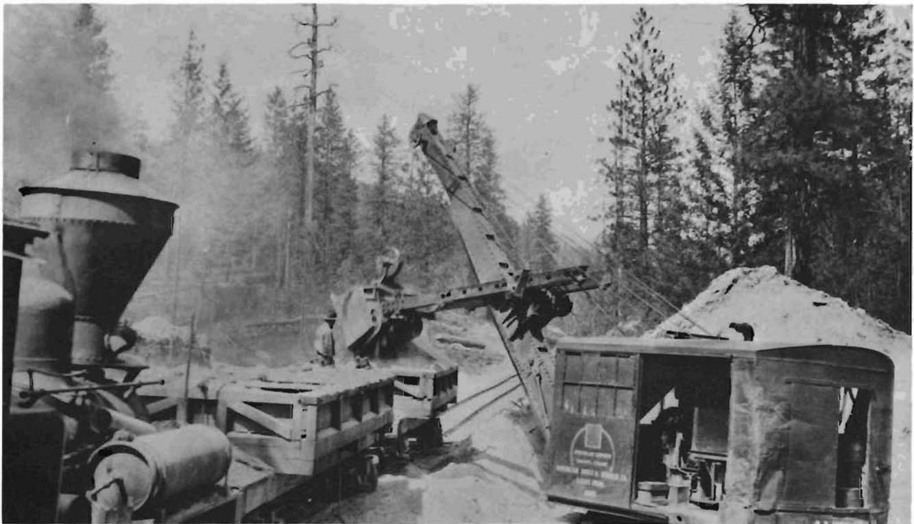
Shay No. 101 and ballast train being loaded by the A. H. & D. "Gopher" shovel on the "C" line in 1929 or 1930. U. S. Indian Service Photo
