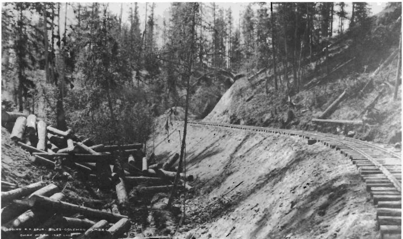
Track of "B" line Southwest of Disautel, Washington, 1927.
