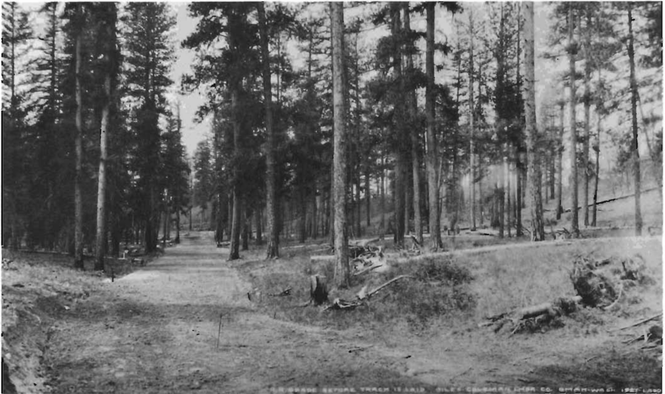
Ladd Photo from E. A. Aston "C" line roadbed ready for the start of track installation in 1927 just to the North of the point where the right-of-way crosses the present route of Washington State Highway 10A.
