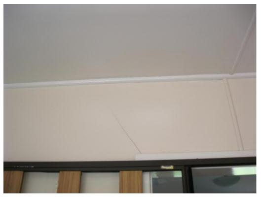
Photograph 6 Cracking to plasterboard linings.
