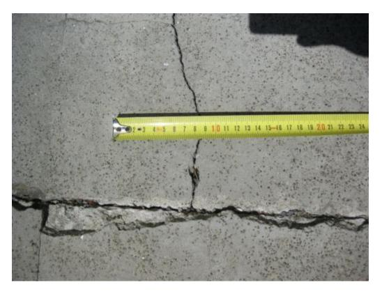
Photograph 5 Cracking to external paving.
