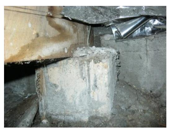
Photograph 7 Timber bearer supported by concrete pile.
