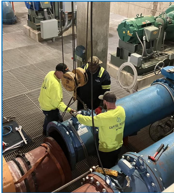
Mag Meter Replacement. Maintenance and Distribution groups were both involved in the project.
