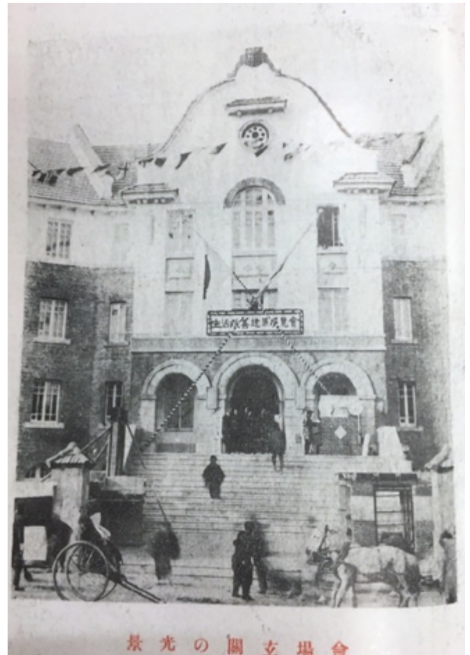
Fig. 2. Photo of the entrance of the Architectural Exhibition of Daily Life Reform held at the SMRC dormitory, Dalian 1921. Published in Manshu Kenchiku Zasshi 1, no. 8 (1921).
