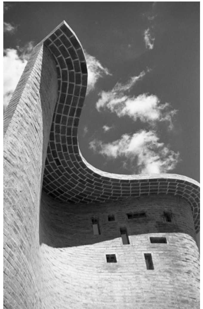
Fig. 1. Church of Christ the Worker, Atlántida, Uruguay, 1958. Detail of the eave that absorbs the thrust of the roof vault and sinusoidal lateral wall. Dieste & Montañez S.A. Photographic Archive, Dieste Foundation.
