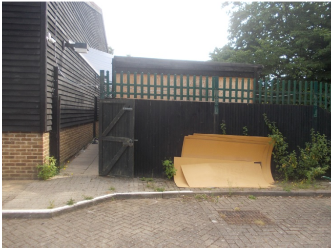
1.Outbuilding with covered walkway
