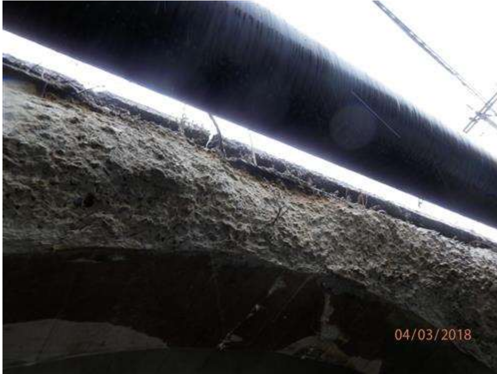
Span 1 east fascia arch exhibits heavy deterioration and spalls with exposed rebar.
