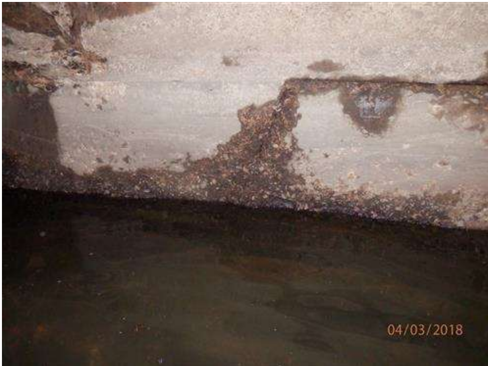
Abutment 1 stem with heavy scale in tidal zone.
