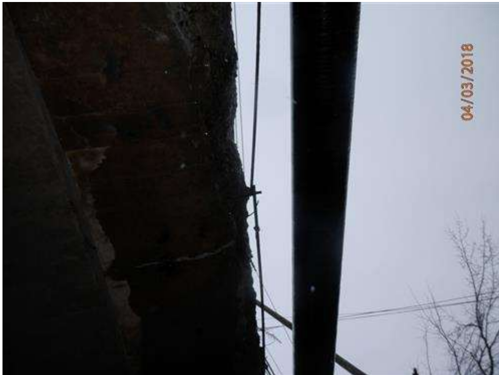
Underside of span 1 east fascia. revealing spalls and exposed rebar.
