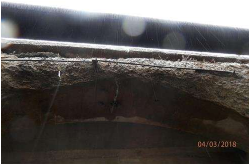
Span 2, east fascia arch exhibiting heavy scale with hollow areas and exposed rebar.
