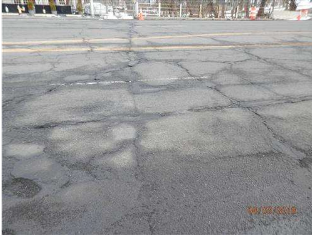
Top of deck at abutment joint, looking west. Note potholes and full width cracks.
