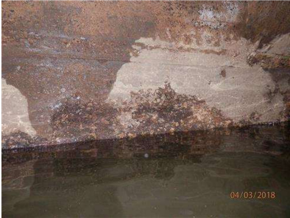
Pier south elevation with heavy scale and spalls in tidal zone.
