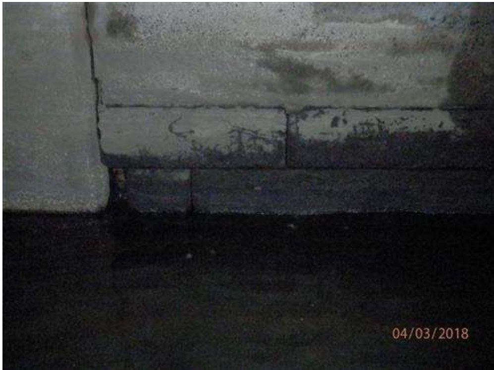
Pier south elevation with void at interface between concrete and masonry sections.
