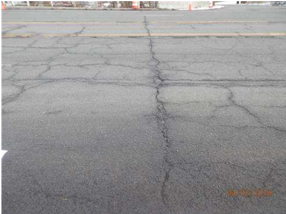
Top of deck at abutment 2 joint, looking west. Note full width crack.
