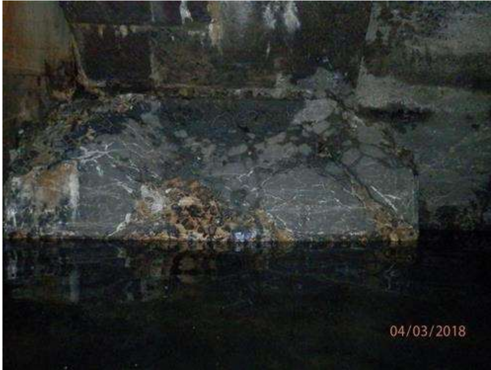
Pier north elevation at arch 2 buttress with heavy scale.
