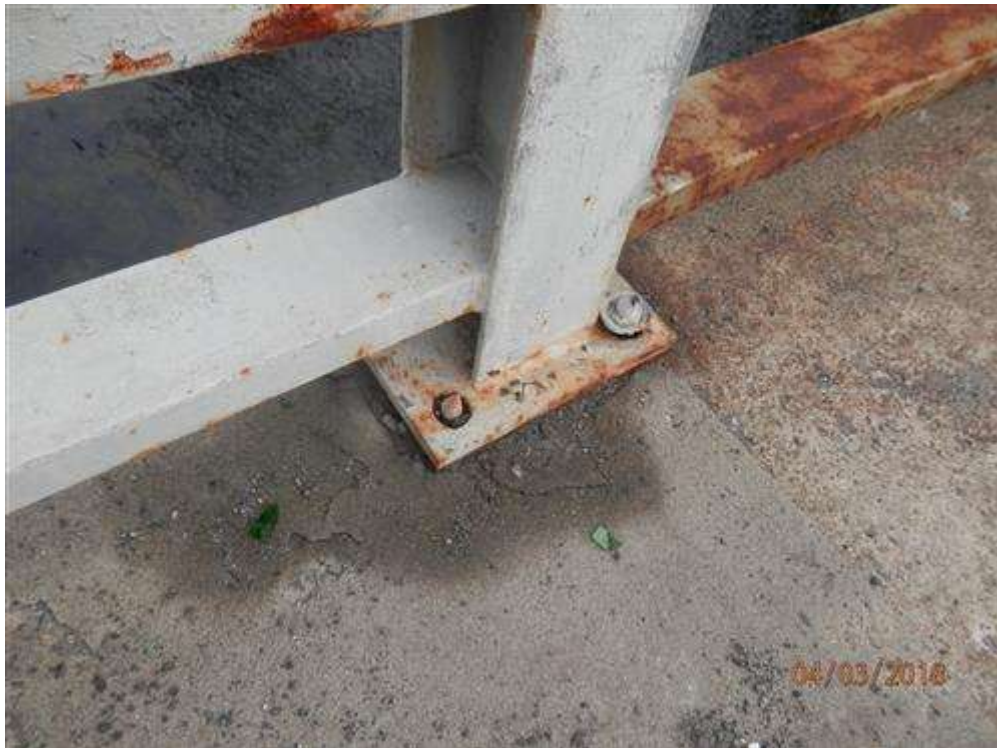
West bridge railing. Note base plate bolt is sheared.
