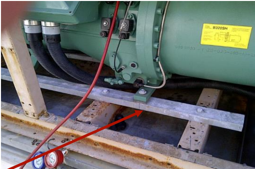
Added "U" Channel for Mounting of the CSH Bitzer Screw Compressor
