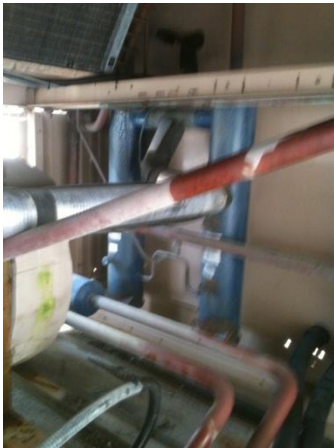
Preparing for External Oil Separator Removal Including removal of the oil line piping and ball valves
