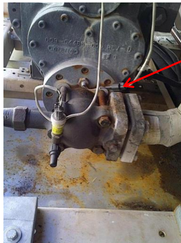
Discharge Temp Sensor
