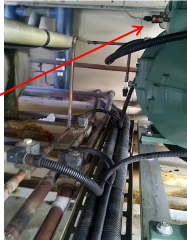
Oil Pressure Transducer
