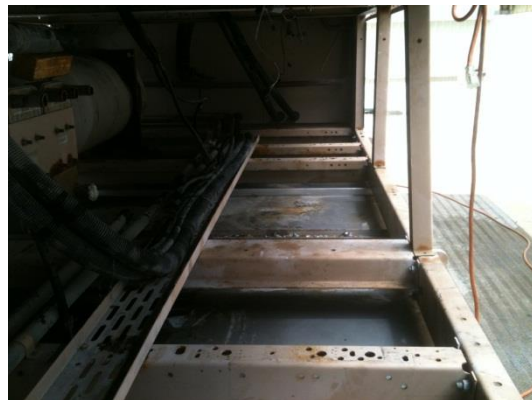
Base Frame cleaned and prepped for installation of BITZER CSH screws
