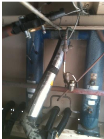
Preparing for External Oil Separator Removal Including removal of the oil line piping and ball valves
