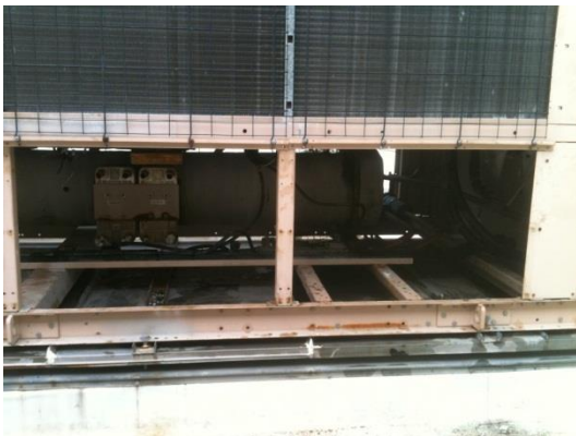
Base Frame cleaned and prepped for installation of BITZER CSH screws
