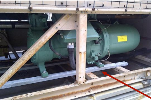
Added "U" Channel for Mounting of the CSH Bitzer Screw Compressor
