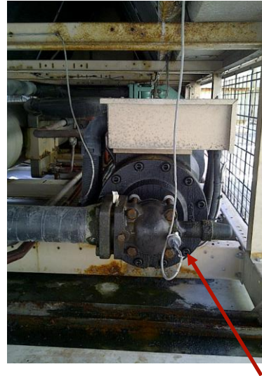
Suction Pressure Transducer
