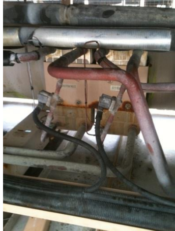
Economizer Heat Exchanger, Thermal Expansion and Solenoid Valve Removal
