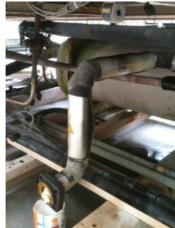
DXS45 compressors removed with existing suction and discharge piping shown
