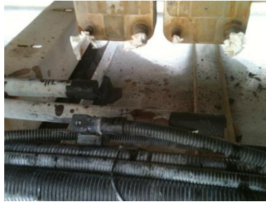
Economizer Heat Exchanger, Thermal Expansion and Solenoid Valve Removal
