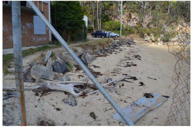
Figure 12 The old cannery building is built on levelled and filled land loosely retained by a derelict rock rubble wall.
