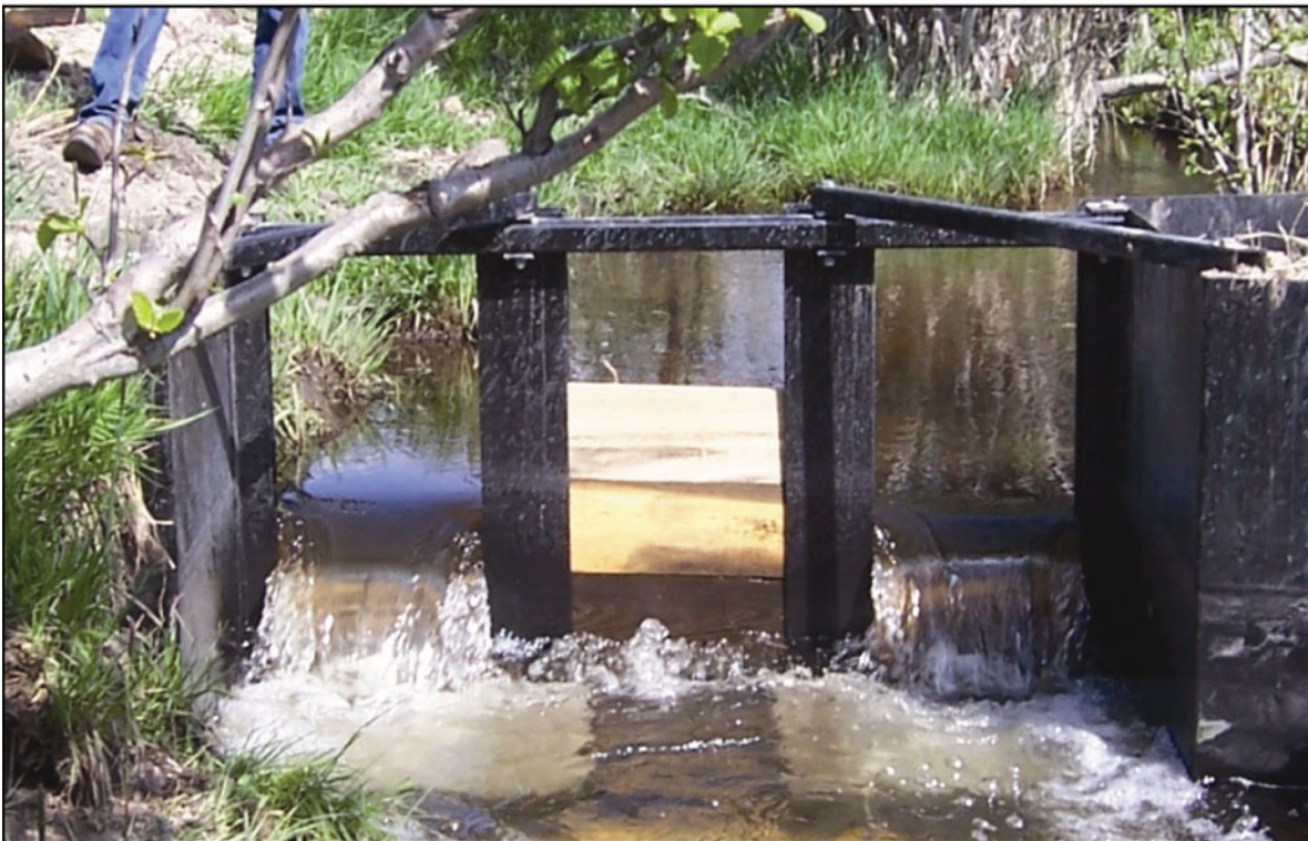
FIGURE 2. Picture of a Coanda diversion and fish screen on Wasson Creek. The photo shows two fish screens as well as a sediment sluice gate (middle slot with boards). The smaller photo (top) shows an adult Westslope Cutthroat Trout ascending the Coanda. (Photo by Jamie Nesbit.)
