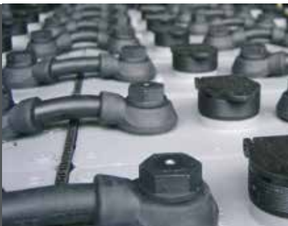
"S-version": the cells are linked by flexible screwed connections.
