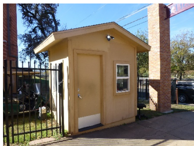
Resource 16 Name: West Security Station Resource Type: Building Stylistic Influence: None Year Built: Unknown Status: Noncontributing Photo(s): 23
