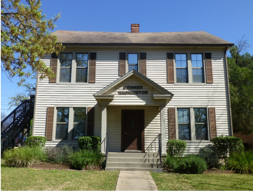
Photo 3: Conner-Washington Building, Huston-Tillotson University, looking east. 3/13/2019.
