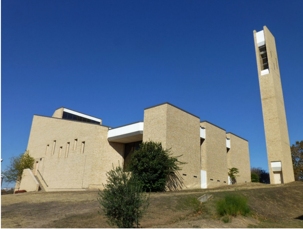
Photo 17: King-Seabrook Chapel and Bell Tower, Huston-Tillotson University, looking north. 12/4/2020.
