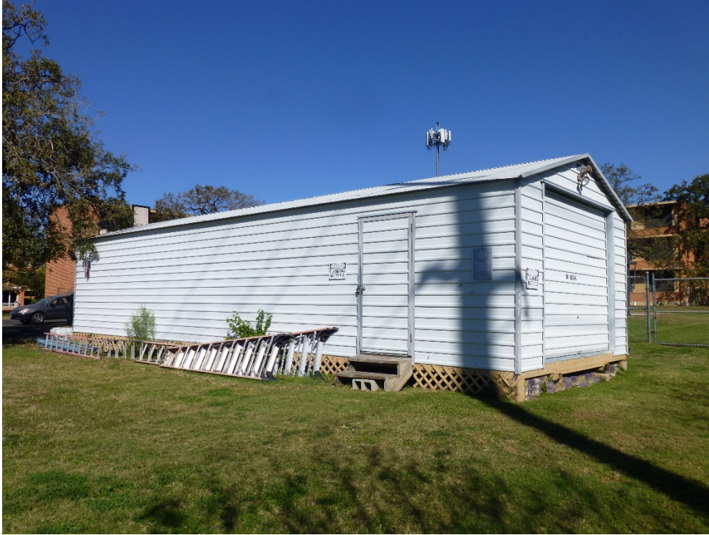
Photo 25: Storage Building (northeast), Huston-Tillotson University, looking northwest. 11/17/2020.
