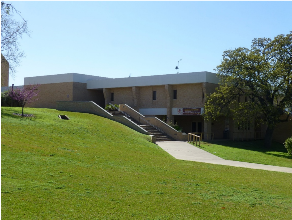
Photo 14: Jackson-Moody Humanities Building, Huston-Tillotson University, looking southwest. 3/13/2019.
