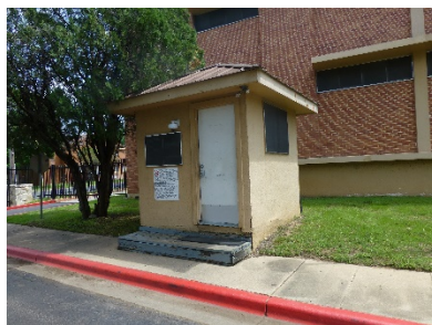
Resource 15 Name: North Security Station Resource Type: Building Stylistic Influence: None Year Built: Unknown Status: Noncontributing Photo(s): 22
