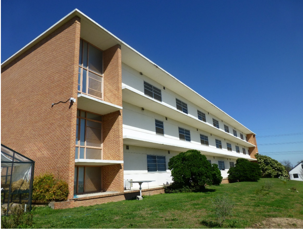
Photo 5: Dickey-Lawless Science Building, Huston-Tillotson University, looking northeast. 3/13/2019.
