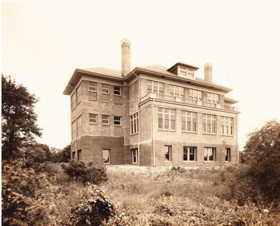
Figure 5: Administration Building (Resource #2). Building File, courtesy Huston-Tillotson University Archives.
