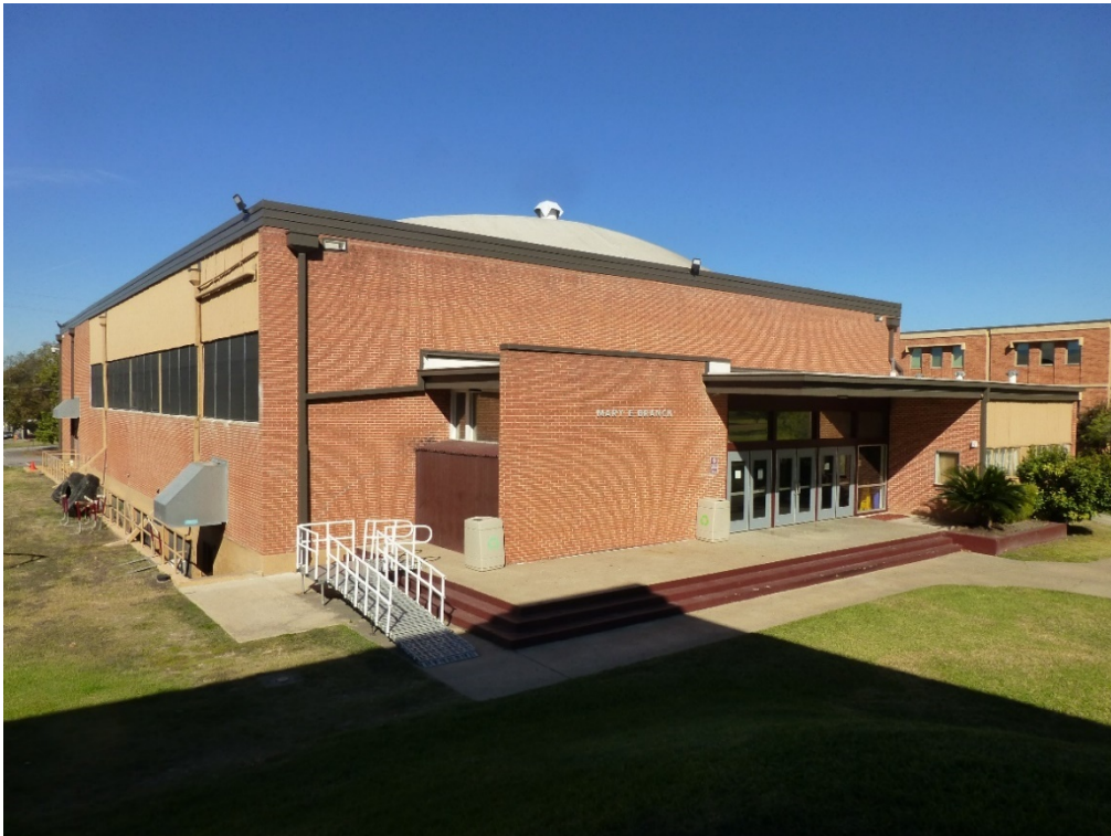
Photo 4: Mary E. Branch Gymnasium and Auditorium, Huston-Tillotson University, looking west. 11/17/2020.
