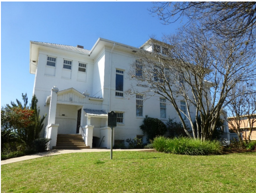
Photo 2: Administration Building, Huston-Tillotson University, looking southeast. 3/13/2019.
