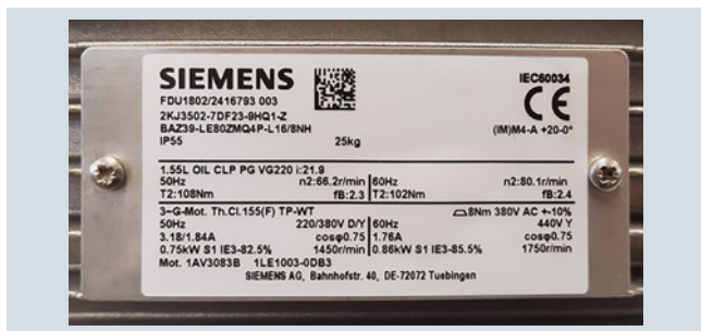
Fig. 12/4 Example, rating plate on the motor
