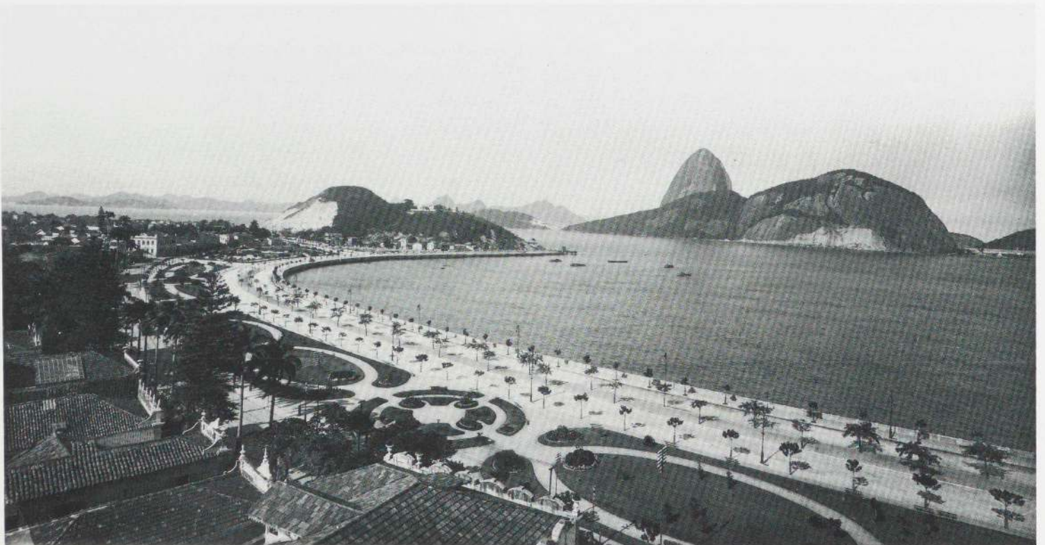
Fig. 14. Avenida Beira Mar, facing Botafogo Bay, Rio de Janeiro. Photograph by Marc Ferrez, 1906
