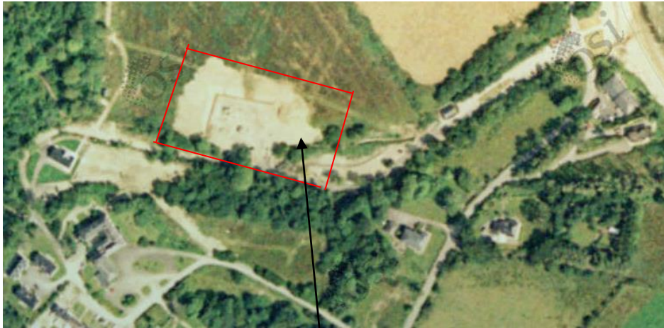
Area proposed for cable landing station
