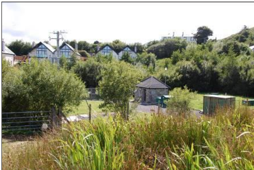
Plate 4 Treatment plant, from north-east.
