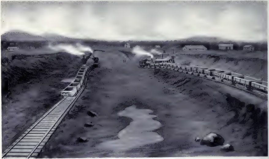
A Typical Michigan Iron Ore Mining Scene
