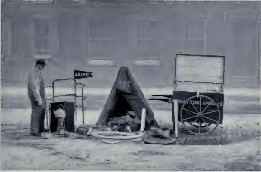
Making Underground Cable Joints in Stormy Weather
