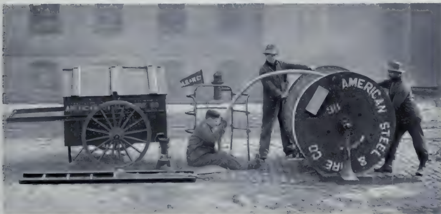
Unreeling Cable into Duct
