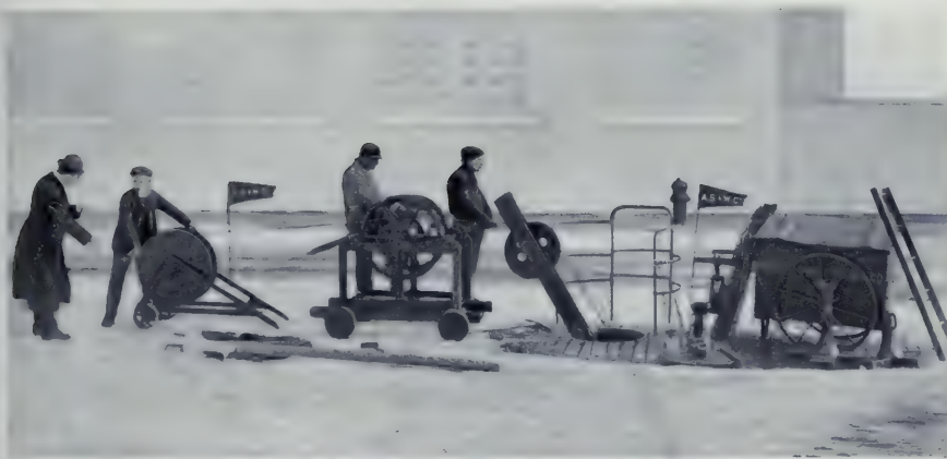
Pulling in Cable with Capstan
