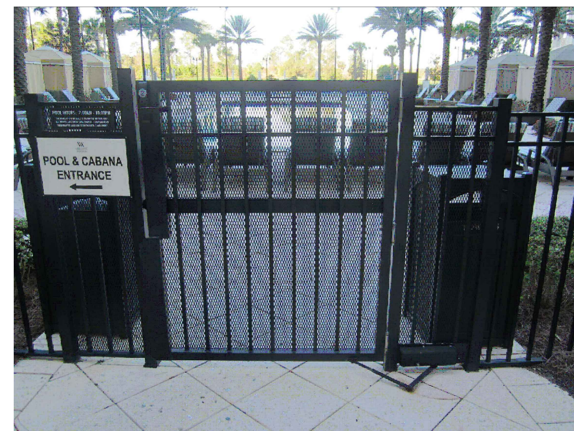
EXAMPLE OF METAL MESH AT GATE
