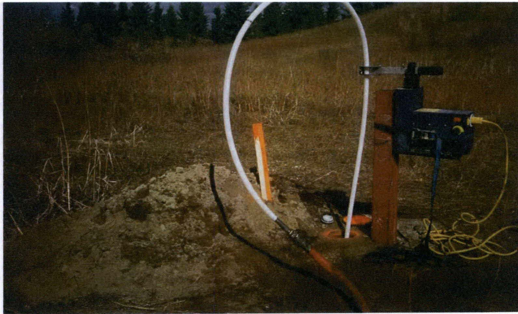
Figure 20. Development of Wells Using Mechanical Waterra Pump
