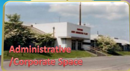
Radford Army Ammo Plant (VA)
