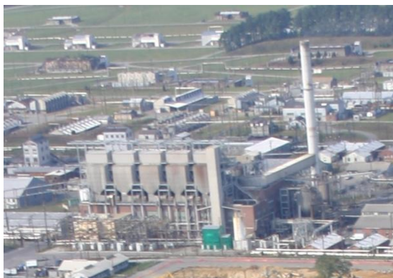
View of Radford AAP Coal Fired Steam Plant
