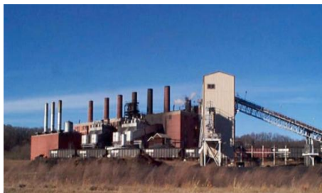
Current Holston AAP Coal Fired Steam Plant
