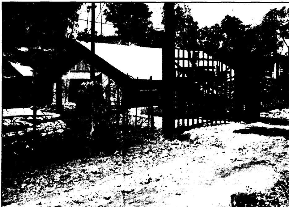
(U) The operations building at Nui Dat
