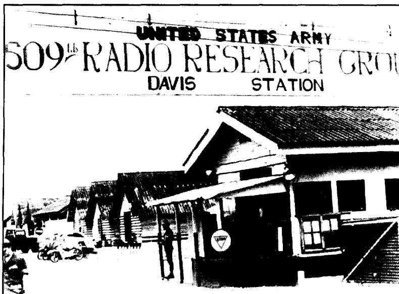
(U) Entrance to Davis Station
