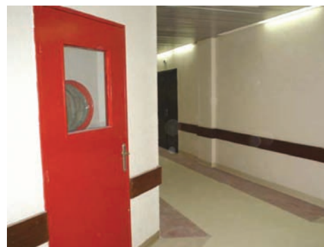
Following renovation, the hallway had a new suspended ceiling and lighting. In addition, walls and door were repaired, and new flooring was installed. (USACE photo, January 8, 2006)
