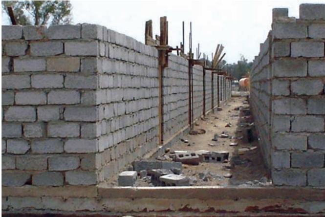
Concrete blocks were used to make load-bearing walls.
