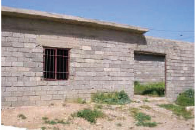
Renovation work included installing a floor, detention cell, and steel bars over windows.
