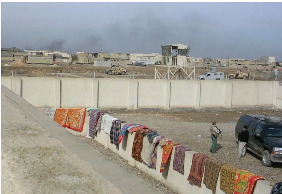
Security fence around police facility.
