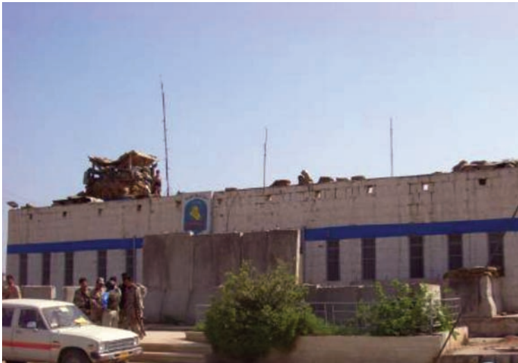
Site before construction: Inadequate guard houses, no security wall, open sewer culverts, and inadequate lighting.
