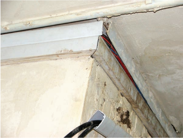
Unprotected high-voltage power cable wires exposed to leaking water.
