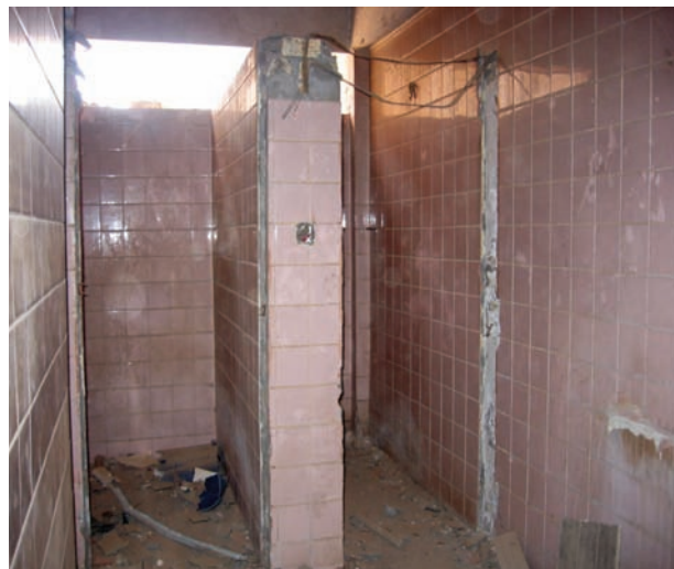
Condition of bathroom prior to renovation.
