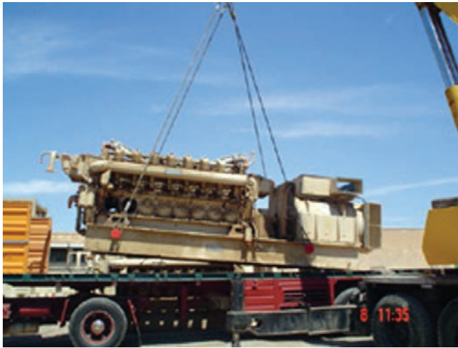
Cockrill generator removal. (Photo provided by USAID)
