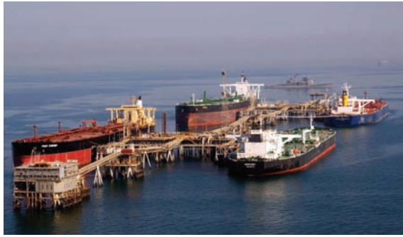
Aerial view of ABOT's four berths. (Photo courtesy of USACE)
