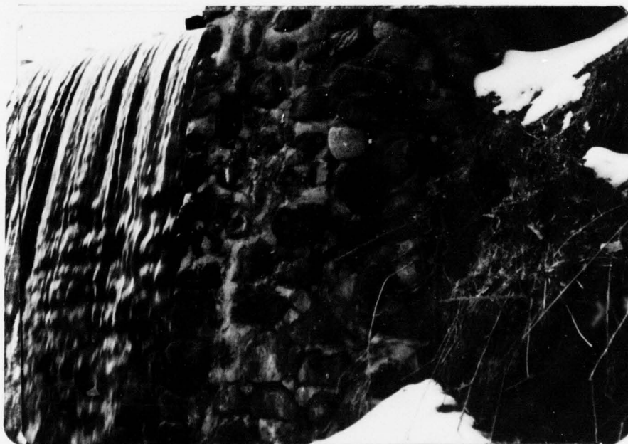
Left retaining wall of spillway. Note replaced cobbles and weep pipe.
