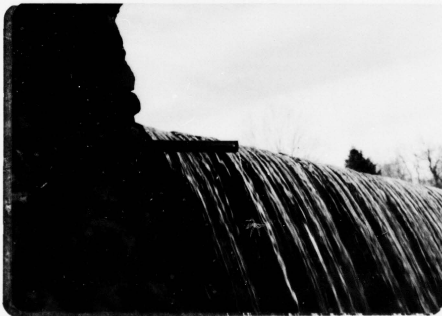
Weep pipe at right spillway retaining wall.
