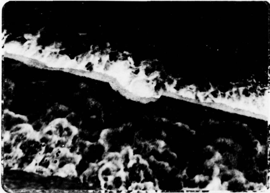
Broken concrete lip of splash bench at toe of spillway.
