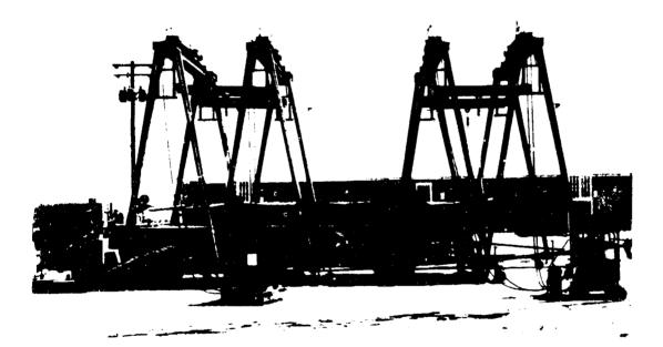
FIGURE 2. C.: gantry system lowering 35,000-pound load onto aircraft loader.
