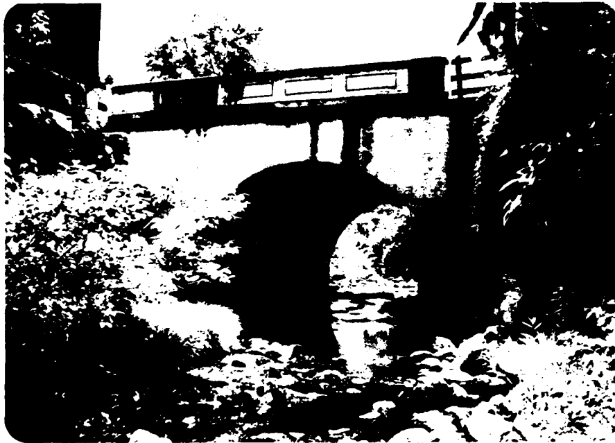
7. View looking downstream of road bridge just below dam
