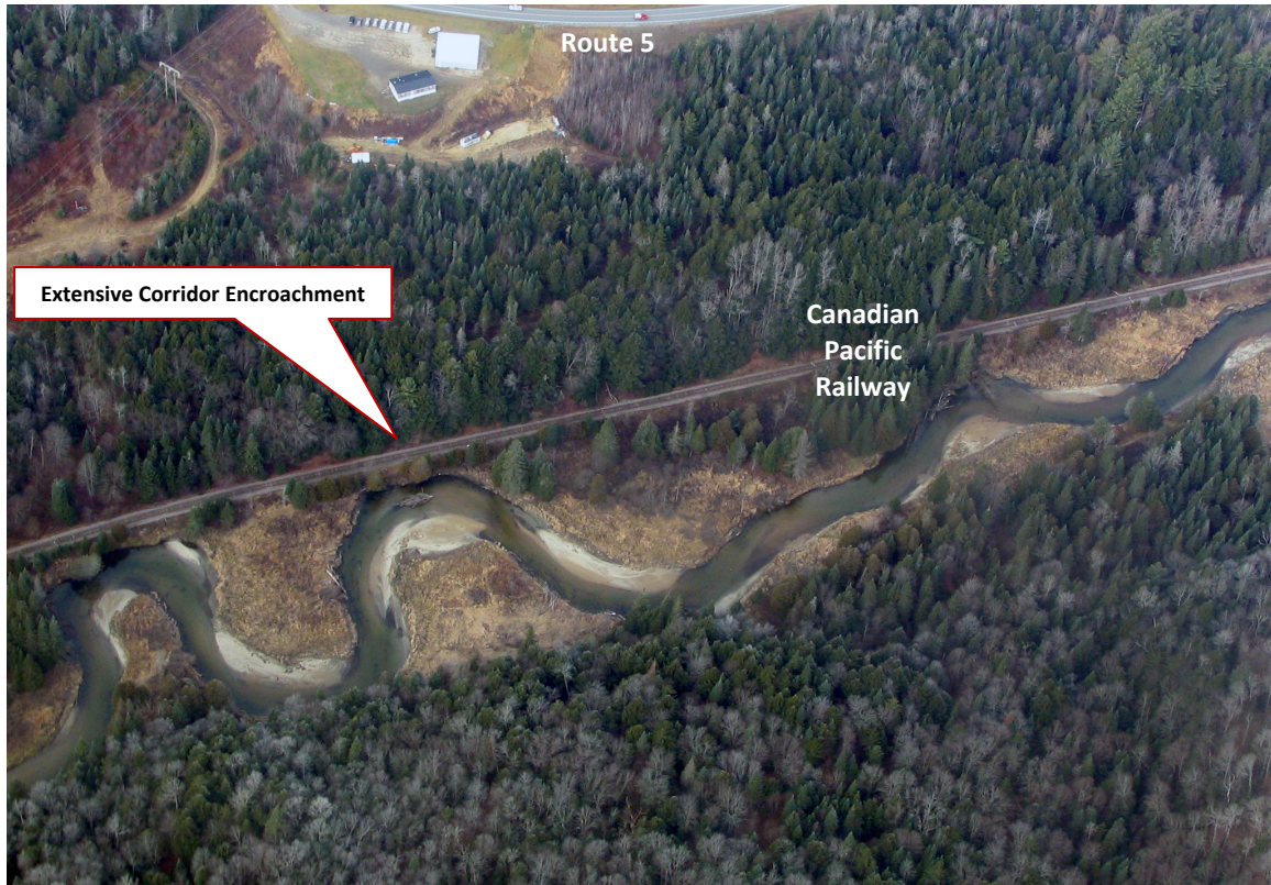
Figure 4.7 Corridor encroachments along the west side of the channel in reach T3.02 and T3.03
