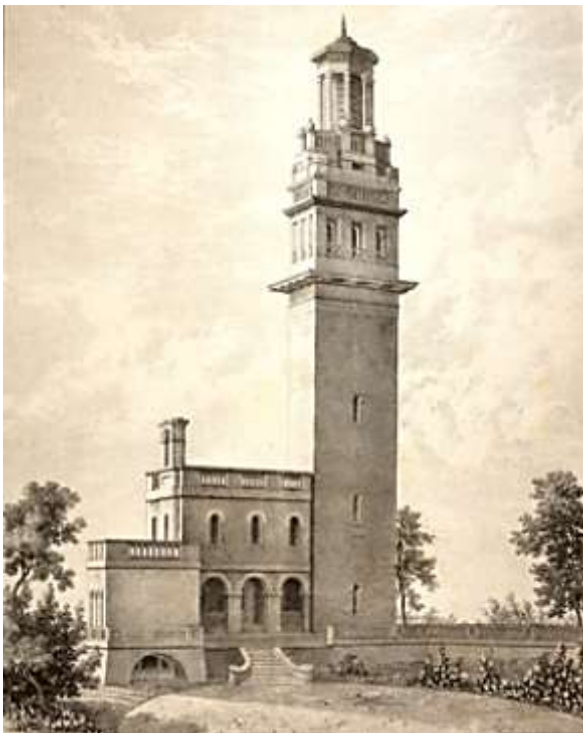
Figure 5 (left): An engraving of Beckford's Tower, viewed from the northeast, illustrates the overall massing scheme of the building. The base is formed of a single story room (left) and a central double story section. The tower is connected to the base at the north corner (right).
