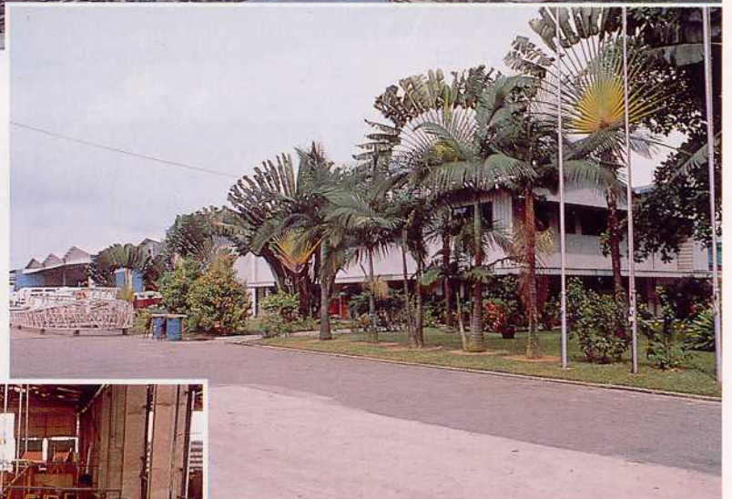
The office area marks the entrance to the yard.
