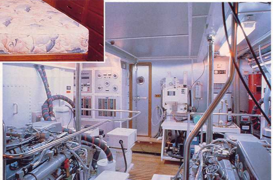
Full width engine room.
