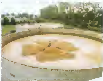
Part of the aerobic biological purification process
