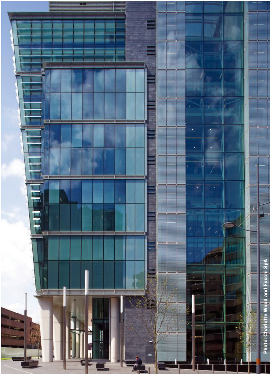
The southwest-facing façade of the Snow Hill station in downtown Birmingham, U.K., is fitted with motor-controlled blinds inserted inside the double glazed unit.
