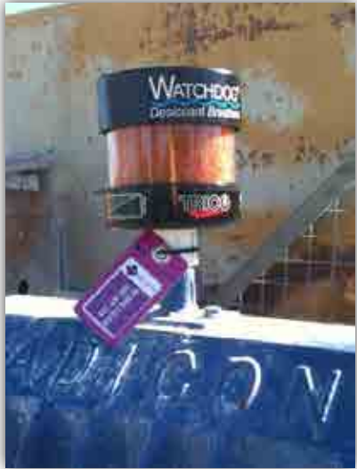
Spectrum Tag on a Watchdog Desiccant Breather
