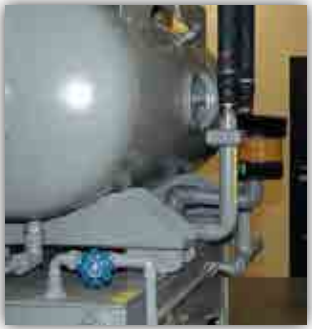
Watchdog Breather installed on a hydraulic reservoir
