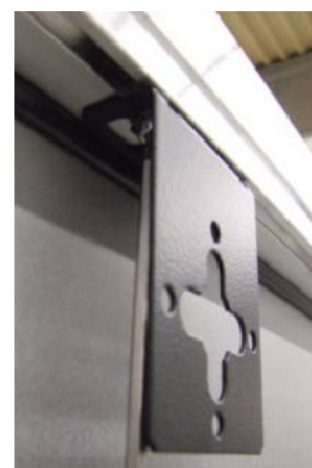
L-Shaped Bracket on Knurr Miracel Horizontal Frame Member
