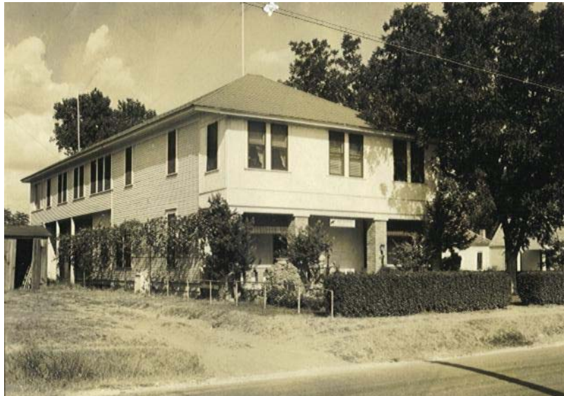
Figure 10: Good Samaritan Hospital, northwest corner, (post-1933 addition).
