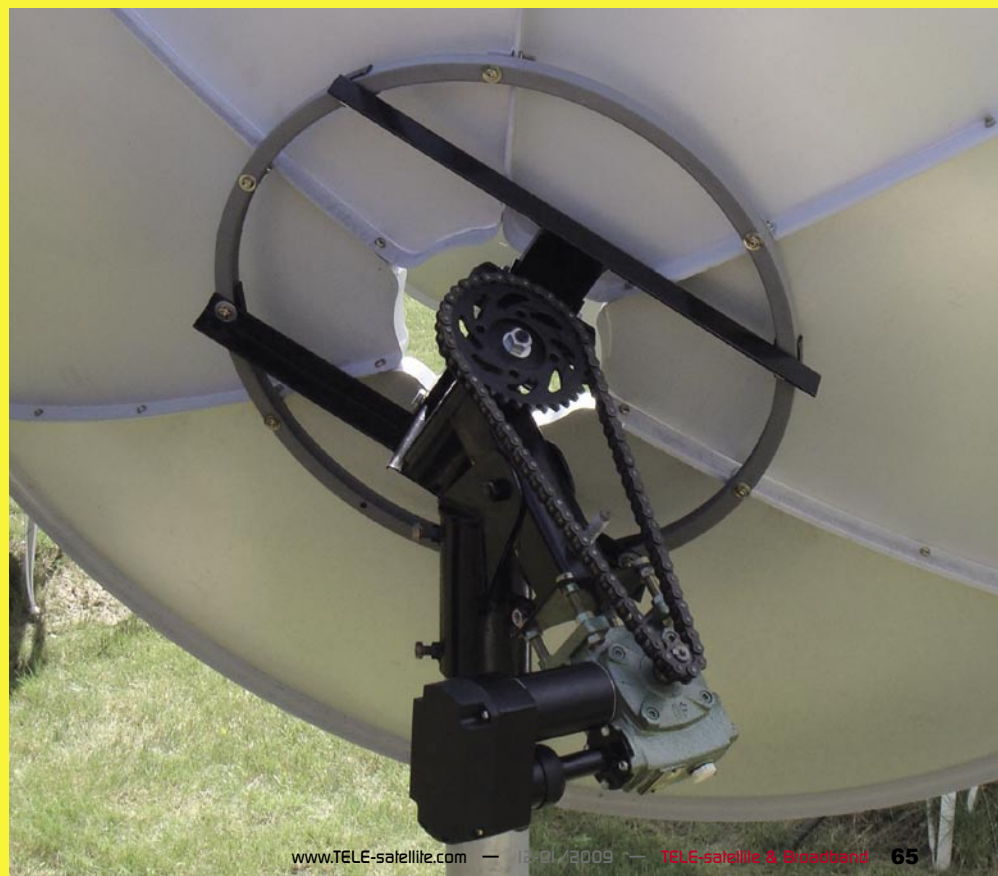
■ Motor from PT. Subur Semesta with chain transmission from the gearbox to the axis
