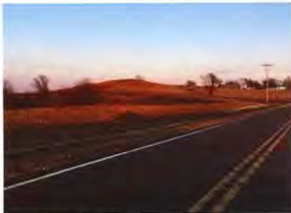
K-4 Highway NE of Dover
