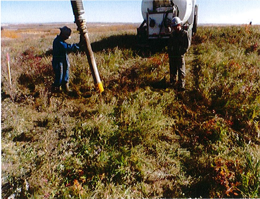
Photo 9: Viewing east toward the Release #4 cleanup.
