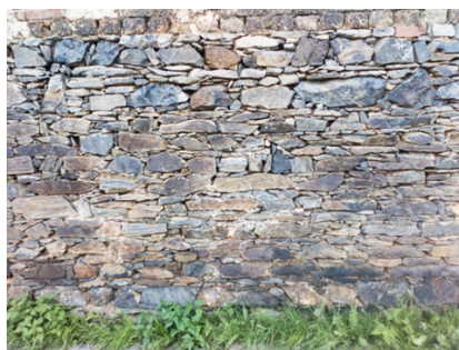
Fig. 3. The wall of residential house, where silicate pieces are combined with adobes. Especially northern walls below slopes had to be reinforced because of abrupt strong floods
