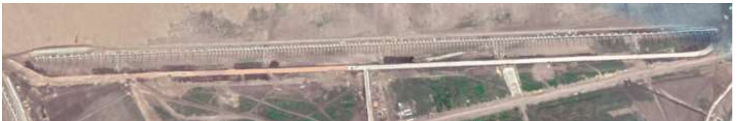
Radar reception site in Kovytkino, Russia © Google Earth
