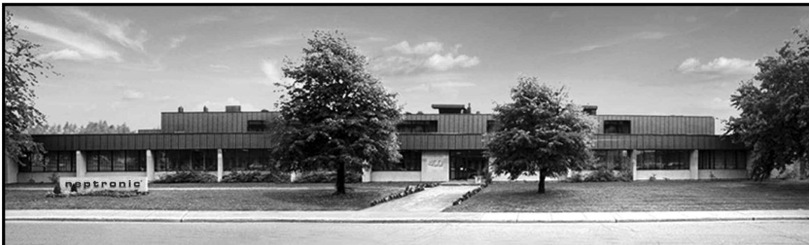
Neptronic headquarters and manufacturing facility Montreal, Canada
