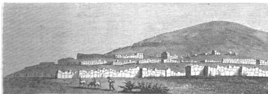
FIG. 4.—REMAINS OF OUTER WALLS OF THE FORTRESS OF CUZCO.
