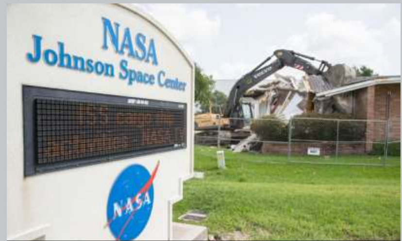
Demolition of Buildings 225 and 226 for New Green Space
