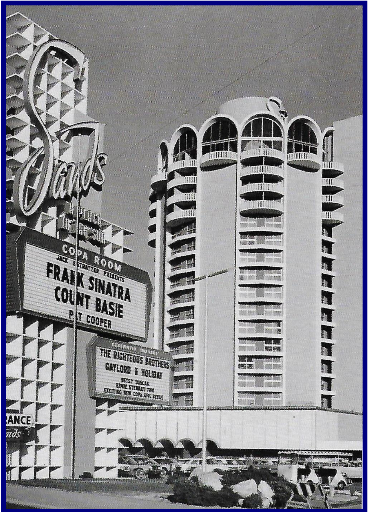
In addition to sunshine, good entertainment and swimming, the Sands even built poolside slot machines and a floating craps table. It was demolished in 1996.
