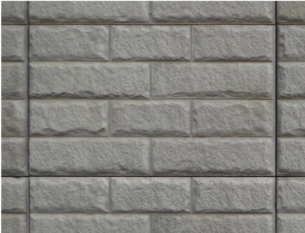
Exhibit C- Gravity Type Precast concrete Units Pattern
