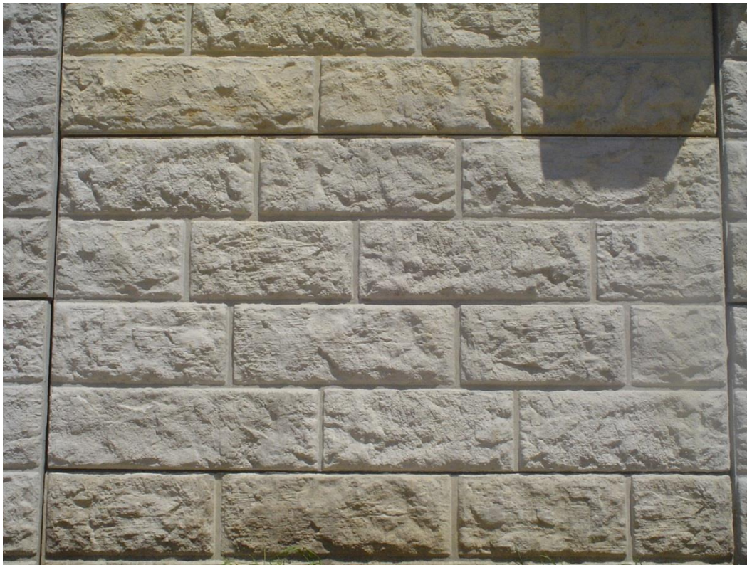
Exhibit B- Precast Concrete Panels Pattern
