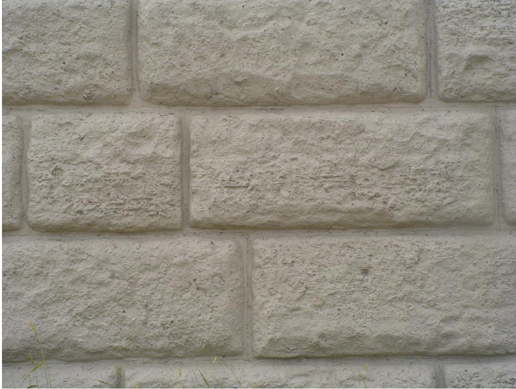
Exhibit A- Cast-in place Pattern
