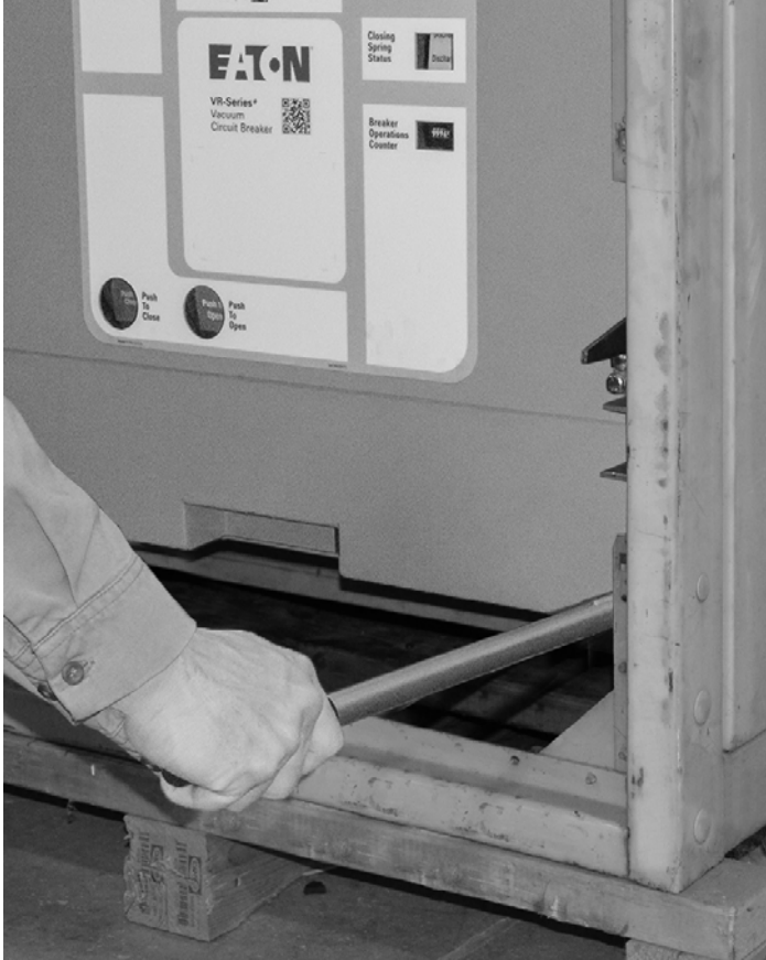
Figure 5.6. Engagement of Secondary Disconnect
