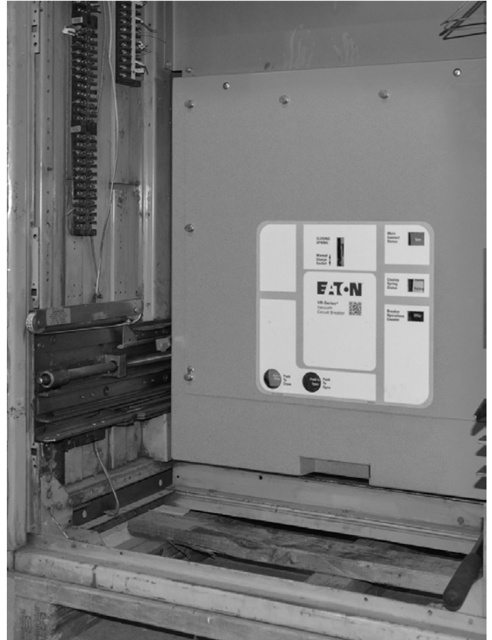
Figure 5.7. VB1-VR+ in the Connect Position
