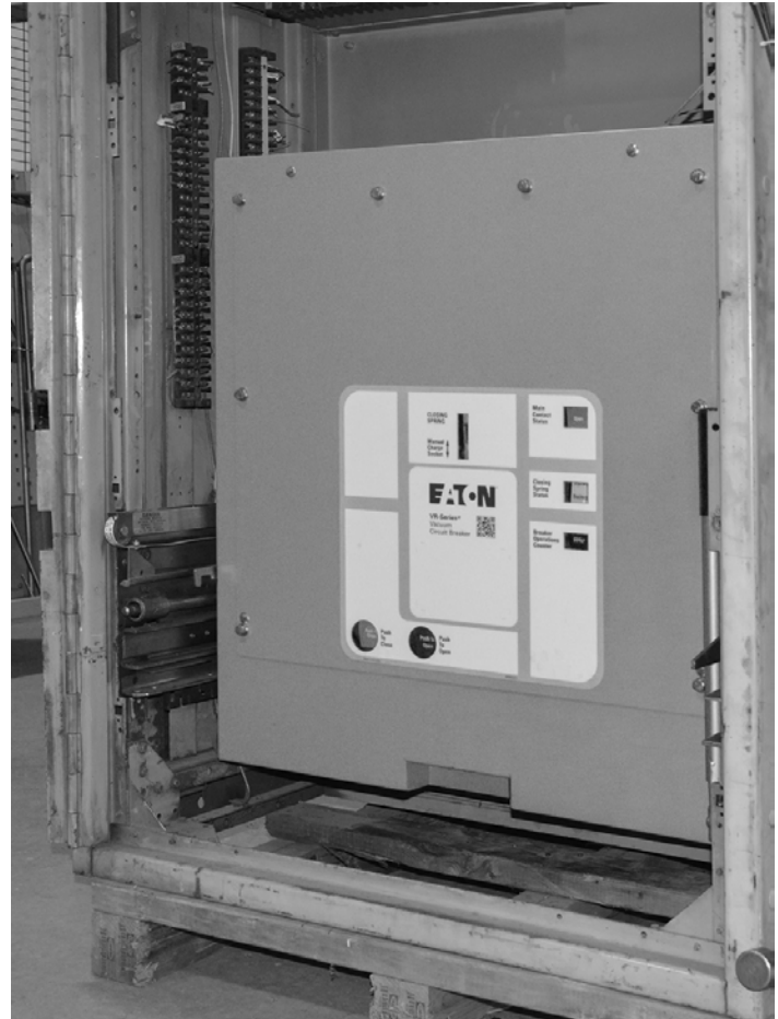
Figure 5.4. VB1-VR+ in the TEST Position
