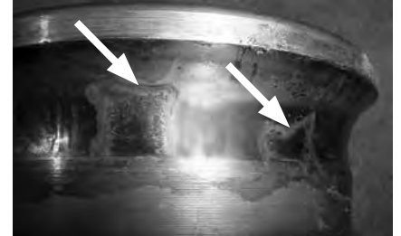
Chemical reaction of grease and moisture in a prolonged static condition resulting in pitting and corrosion. A 'witness mark' is generated at each ball location on the inner race.
