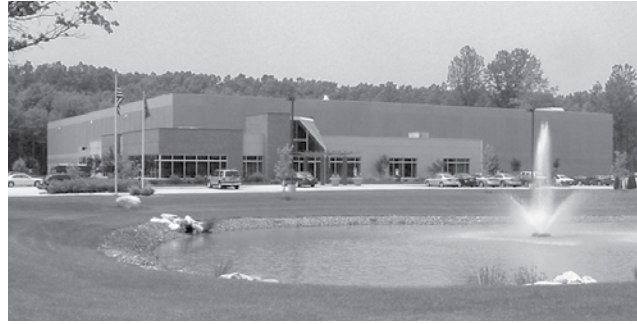
North Coast Bearings services our customers from our 110,000 square foot Avon, Ohio facility along with a distribution center in Sparks, Nevada. The DT Components brand of kits are also available from additional Timken distribution centers throughout the world.
